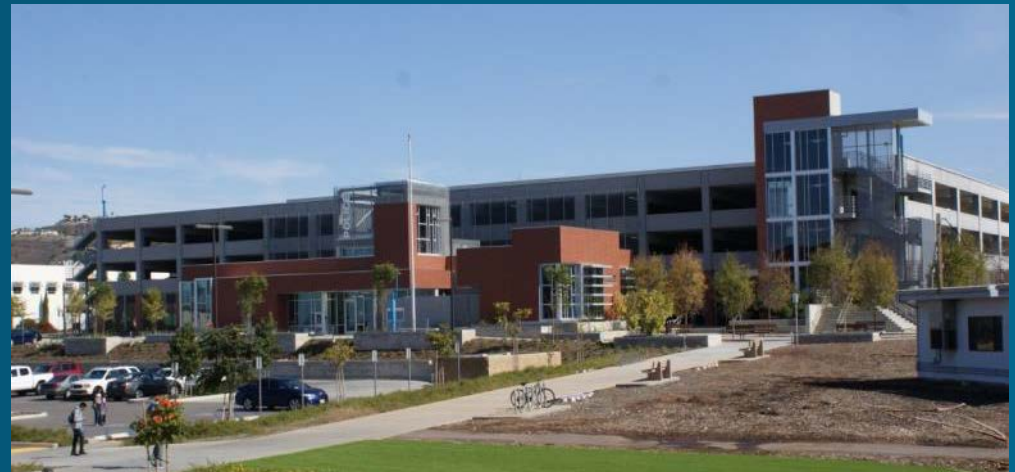
Police Station & Parking Structure
